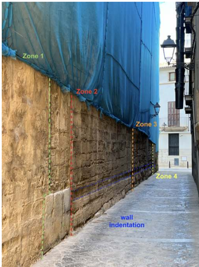
Figure 7. The Eastern Wall on Carrer del Vent with colored demarcations of the construction seams separating the different zones of stonework, Palma de Mallorca (photograph and overlay by the author)
